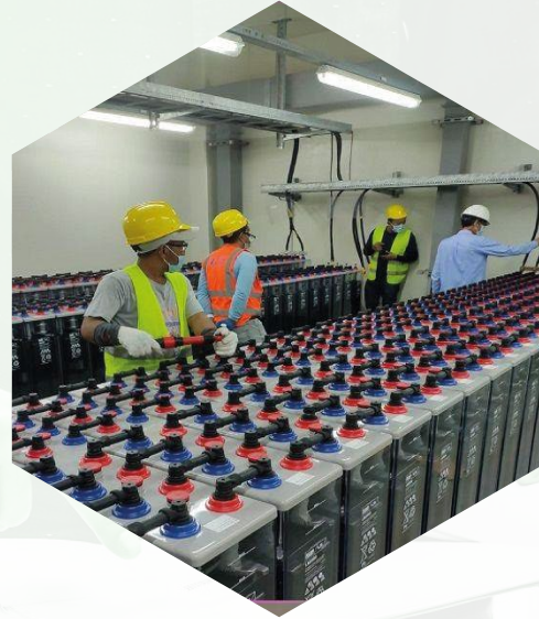
Battery Replacement Client: Shuhaibah Water & Electric Co. (SWEC)
